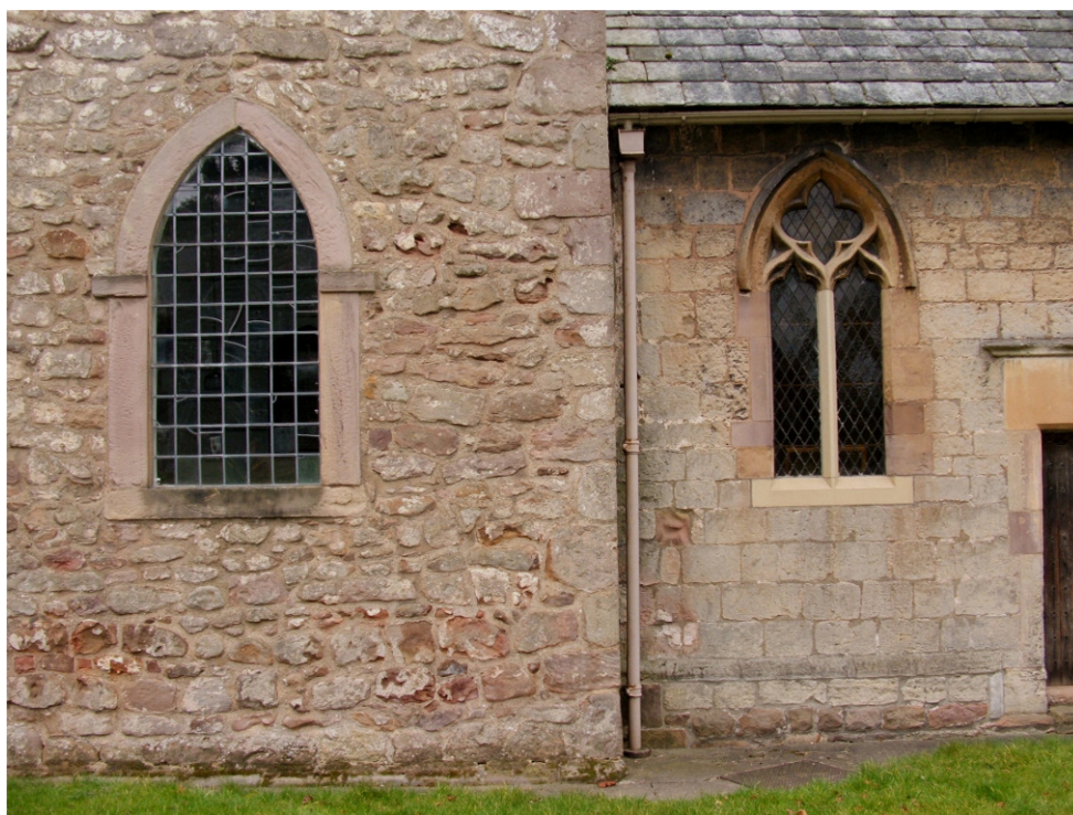
Figure 49: A pre-conquest date has been ascribed to the nave of Todwick church on account of its use of coursed red-sandstone masonry (left) and the survival of typically Saxon ‘side alternating’ quoins at the angle of this wall. Photo by Dan Ratcliffe © SYAS 2005
